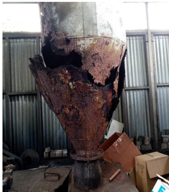
Figure 30: Incinerator in disrepair at Popondetta Provincial Hospital
