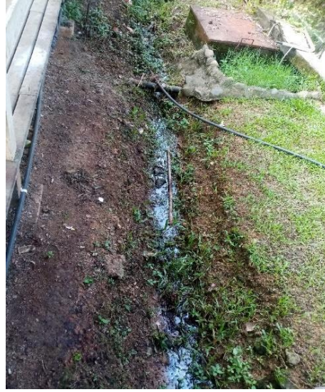
Figure 32: Example of poor drainage at incinerator site
